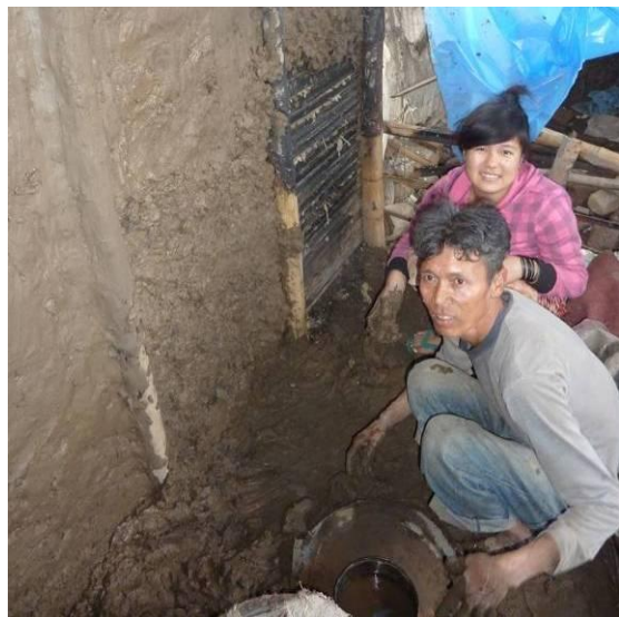
Above: The Tamang family re-building their home in the Kalimati slums after it burnt down in an accidental fire.
